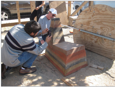
Figure 2. Rammed earth chair constructed at the Barelas Community Gardens.
