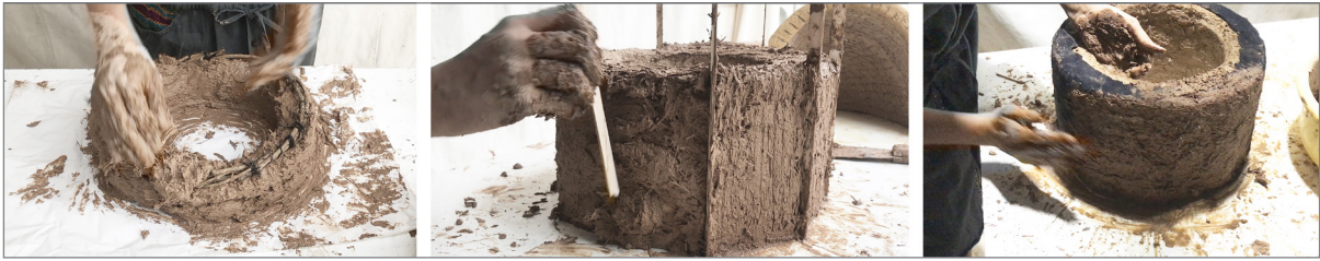
Figure 6-1. Clay Cylinders are made by rounded sticks then filled and shaped by straw and clay. The envelope of the cylinder is screeded to make a round and acceptable base for plastering. Layer of clay plaster is applied adding ochre pigment, and the motif is carved on it by chisels.
