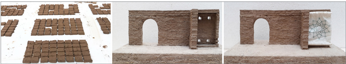
Figure 7. Around 700 miniature adobes are made by each student to make an adobe thermal mass wall. This wall plays a climatic role as a thermal mass; like a part of a Tromb wall or a wind catcher. During this project students learn the techniques of masonry and also plastering.
