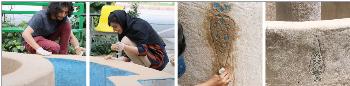
Figure 5. Lime plaster of the pool. After curving the motifs, milk is applied to make a more resistant plaster.
